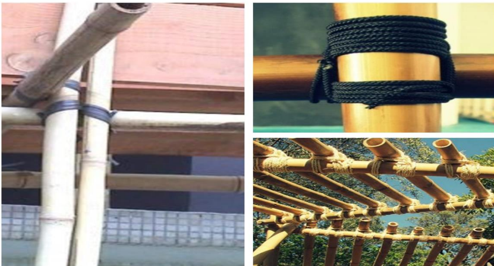
Fig. 3. Lashing joint [44]
