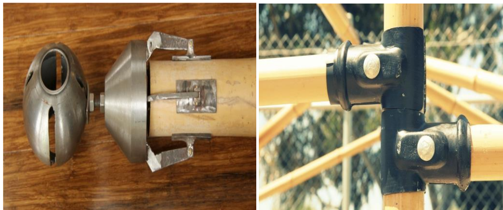
Fig. 8. Clamp Connectors for bamboo [15]
