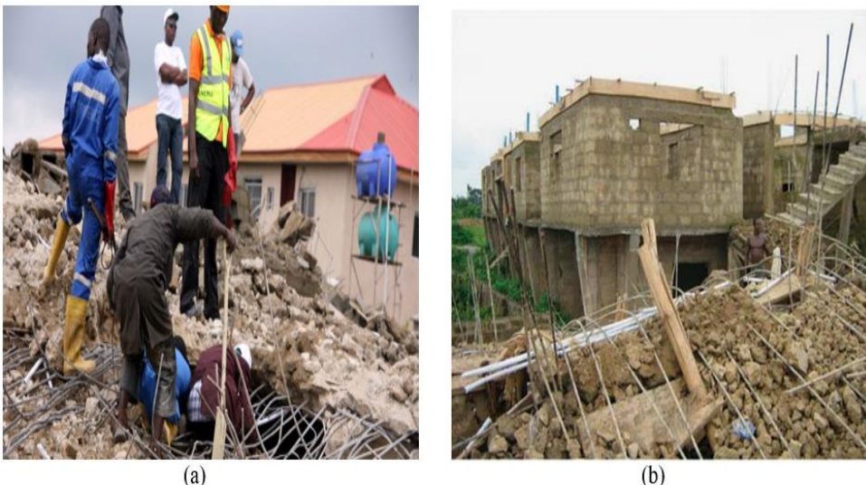
Fig. 1. Sample images of building collapse caused by different variables, (a) building collapse in Federal Capital Territory, Abuja [8], and (b) building collapse in Ondo State as a result of substandard materials [9]
