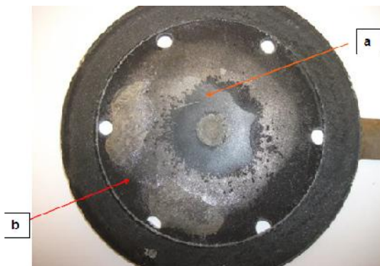
Fig.11. The coated test plates after two months of exposure to geothermal steam. Central the eroded area (a) and scaling deposition from the geothermal steam (b).
