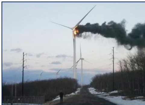
Fig. 2. Wind turbine fire - Locust Ridge Wind Farm, USA 2 [7]
