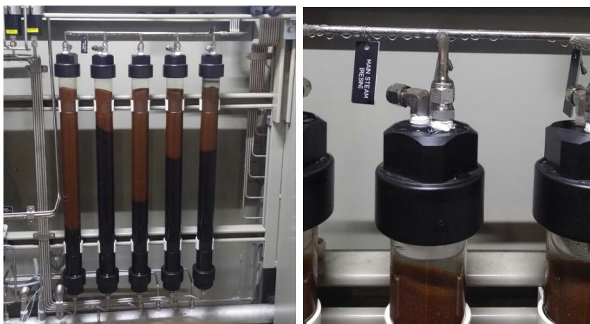
Fig. 3. Power plant's on-site photo of the column
